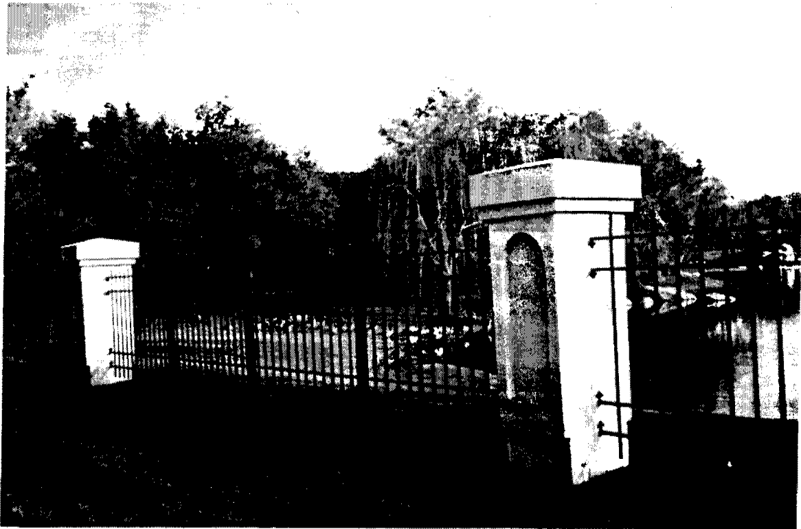
▶ SPIKE TIPPED WROUGHT IRON - DANGEROUS TO WILDLIFE
