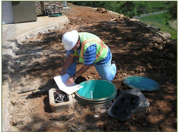
Figure 11.1.2: A County worker inspects a new septic tank effluent pumping system.
