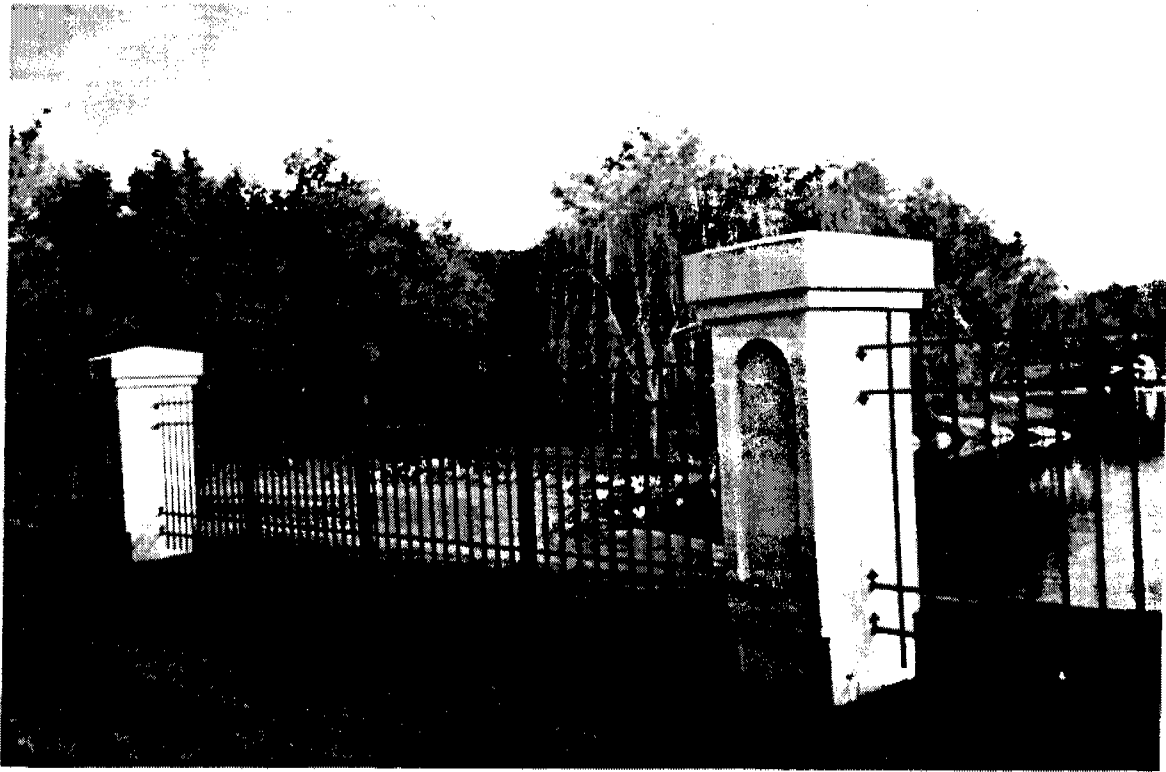
▶ SPIKE TIPPED WROUGHT IRON - DANGEROUS TO WILDLIFE
