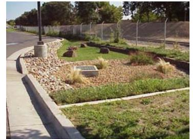
A sand filter is a two-stage constructed treatment system including a pretreatment sedimentation basin and a filtration basin containing sand.
