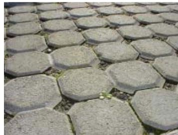
Porous pavement allows stormwater runoff to infiltrate into the ground through voids in the pavement materials.
