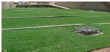
A Vegetated Filter Strip is a gently sloped soil surface planted with dense, sod-forming vegetation and designed to receive and treat sheet flow runoff from adjacent surfaces.
