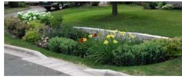
A stormwater planter is a low-lying vegetated planter that receives runoff from roof drains or adjoining paved areas. A shallow surcharge zone above the vegetated surface temporarily stores stormwater.
