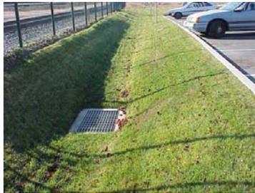
A vegetated swale is a wide, shallow, open channel planted with dense, sod-forming vegetation and designed to accept runoff from adjacent surfaces.
