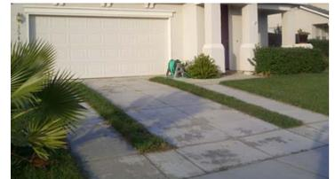
Alternative driveways exhibit one or more of these features: they have permeable surfaces, drain to landscaping, provide access to more than one house, and/or limit concrete use to narrow driving strips.
