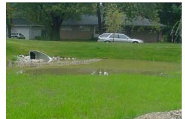
An infiltration basin is a shallow earthen basin constructed in naturally pervious soils and designed for infiltrating stormwater.
