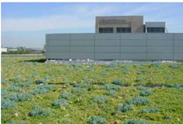
A green roof is a multi-layered, vegetated rooftop system designed for filtering, absorbing, and retaining stormwater.
