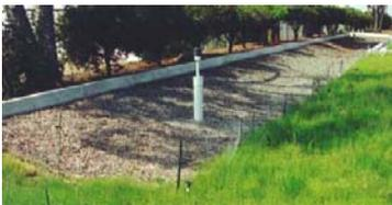
An infiltration trench is a long, narrow trench constructed in naturally pervious soils and filled with gravel.
