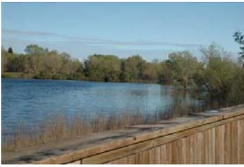
A constructed wetland basin is an earthen basin treatment system with a permanent pool of water. The basin contains an area above the permanent pool to retain runoff from the stormwater quality design storm and slowly releases excess water over a specified drawdown period.
