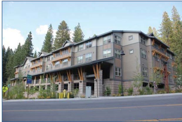
New Housing in Kings Beach
