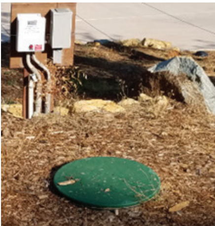
Typical STEP system control panel and lid
