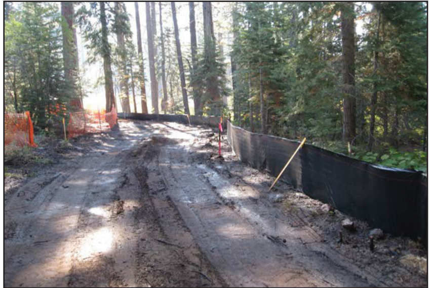
Tree protection during construction Photo Source: CDM Smith
