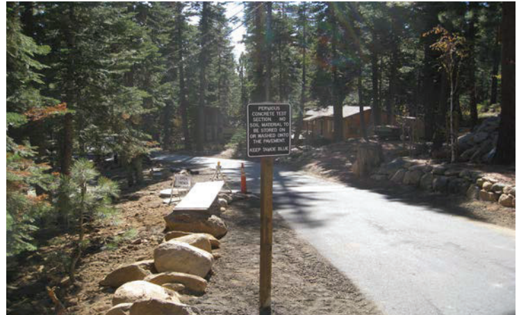
Pervious Concrete road in North Lake Tahoe, Placer County. Source: CDM Smith
