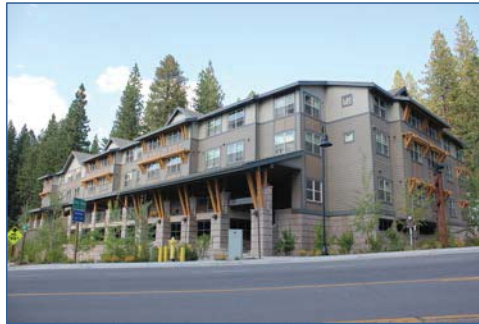
New Housing in Kings Beach
