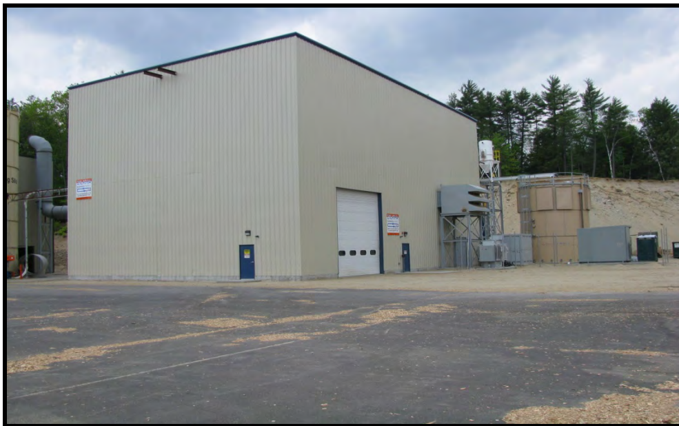
Exhibit 3-5: Zilkha Installation in New Hampshire
