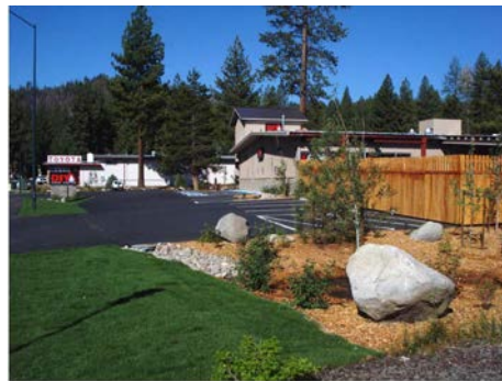
Ensure that loading areas do not interfere with other site circulation, and permit free use of aisles, driveways, and sidewalks during freight operations.
